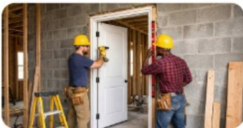
DOOR FRAME FIXING
