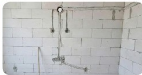
CONDUITING IN THE BLOCKS MASONRY
