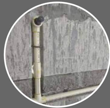
CONDUITING IN THE BLOCKS MASONRY
